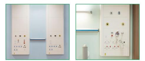
Electrical sockets are fitted and can be fully wired and tested with essential/non essential sockets available for standard ward areas and blue isolated earth sockets for A&E, critical care or operating departments. Medical gas terminal units from all manufacturers can either be provided as a fully pregassed and tested system or alternatively, mounting provision can be included for installation on site.
